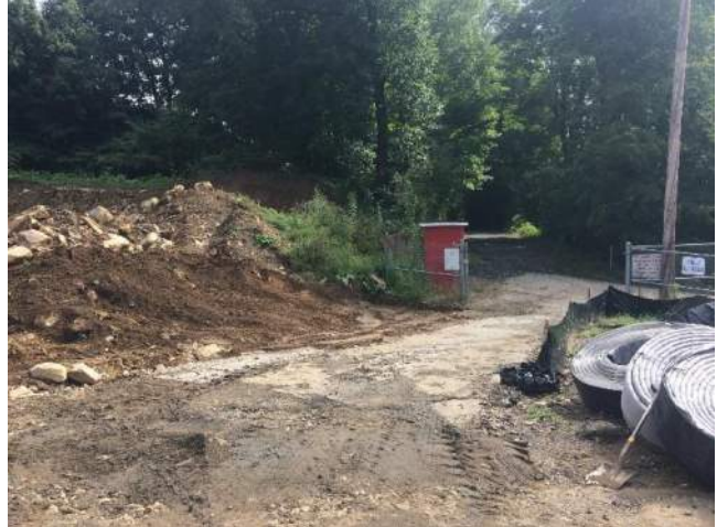
Repairs at South Construction Entrance.
