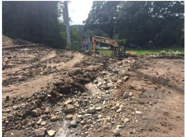
Erosion Gully West at V. Bleachers
