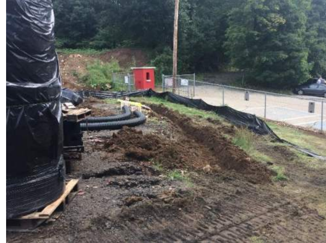
Repairs at South of Track
